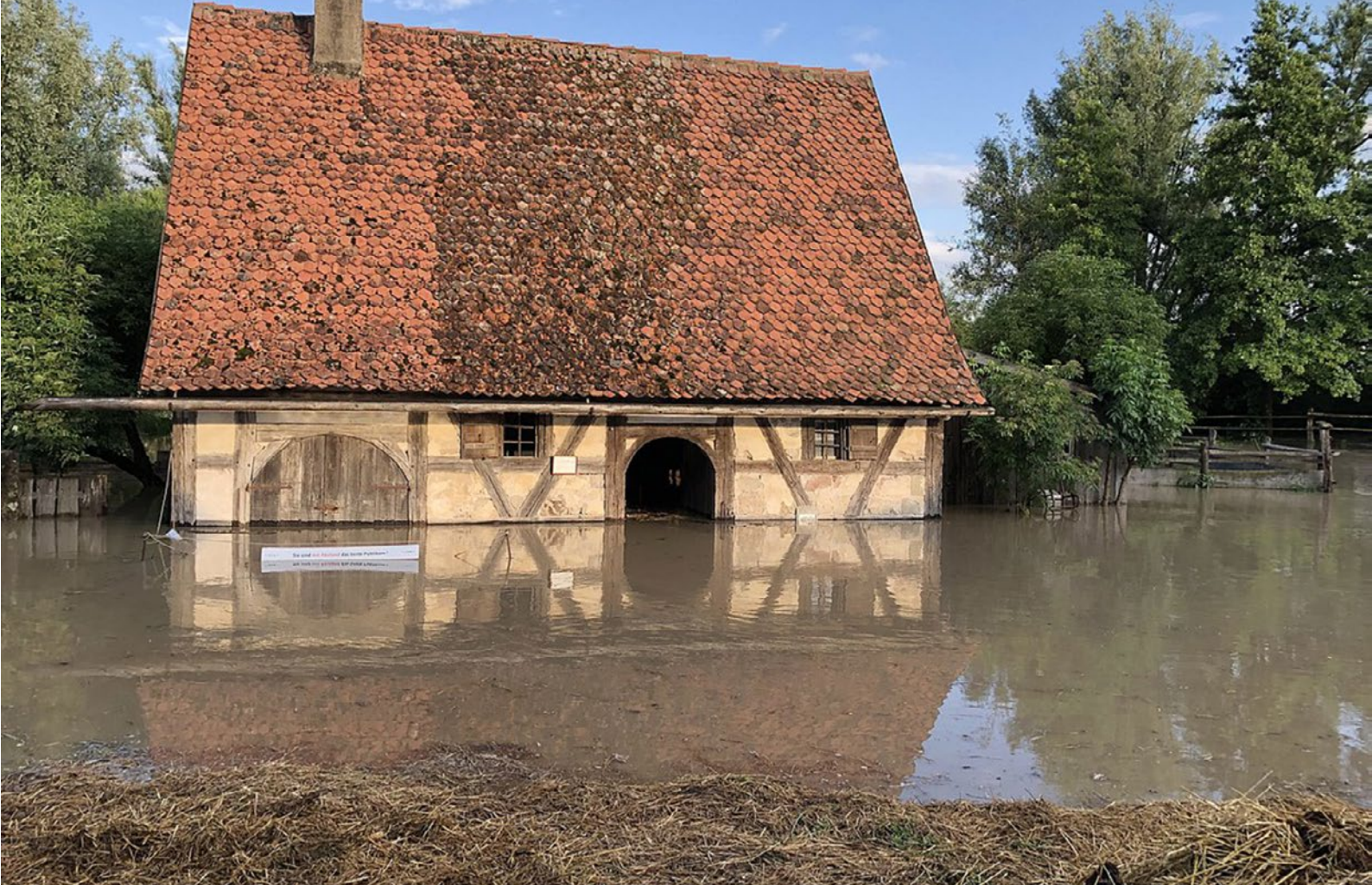
Half-timbered building in Bad Windsheim (Germany) after extreme rainfall on July 15, 2021 © Freilandmuseum Bad Windsheim
