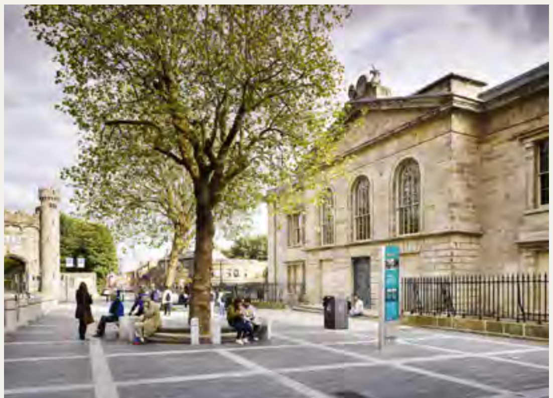
Kilmainham Courthouse, Dublin, adaptation and reuse by OPW Architectural Services. RIAI Award winner, 2017. Photo by Ros Kavanagh.
