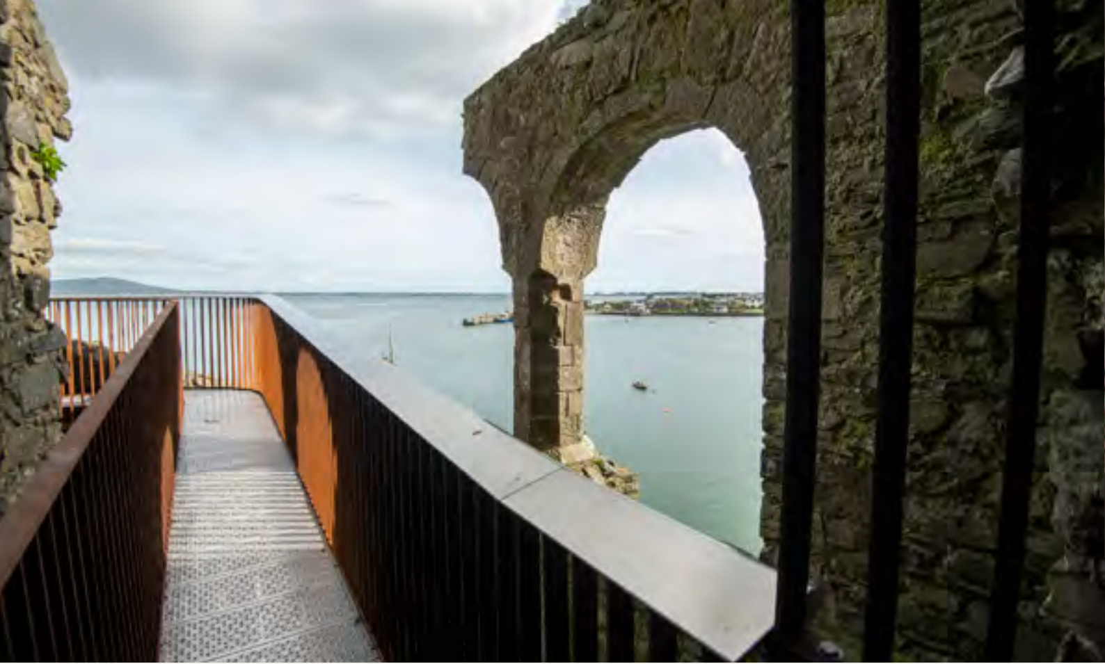
Carlingford Castle, County Louth, interventions by Howley Hayes Architects. RIAI Award winner, 2021. Photo by John Lalor, National Monuments Service, DHLGH.
