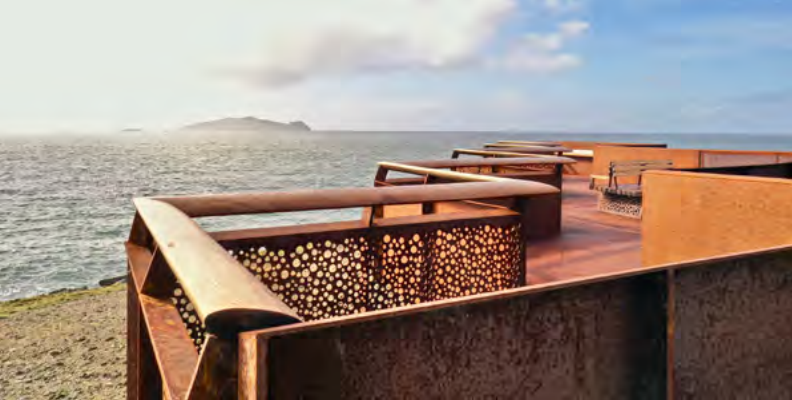
Wild Atlantic Way Viewpoint, Co Kerry by Paul Arnold Architects. RIAI Award winner 2021. Photo by Lorcán Ó Cinnéide.
